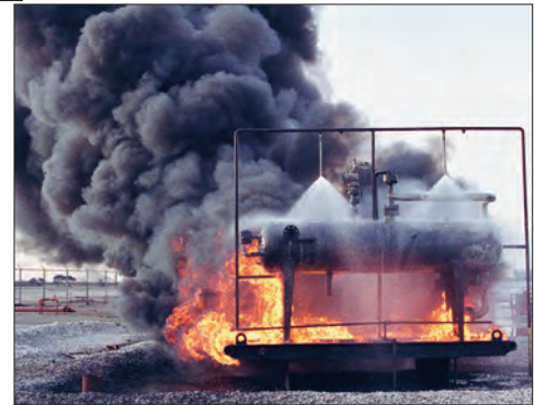
N6 nozzles protect a propane storage tank from fire and explosion.
